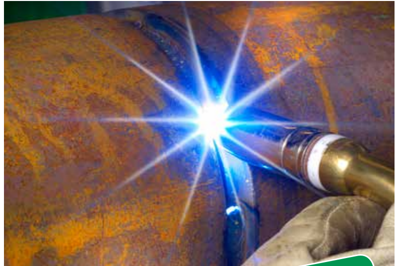
IAC™ - Vertical downwards welding of a root pass in a district heating pipe. Welding speed is significantly increased compared to traditional upwards welding..
